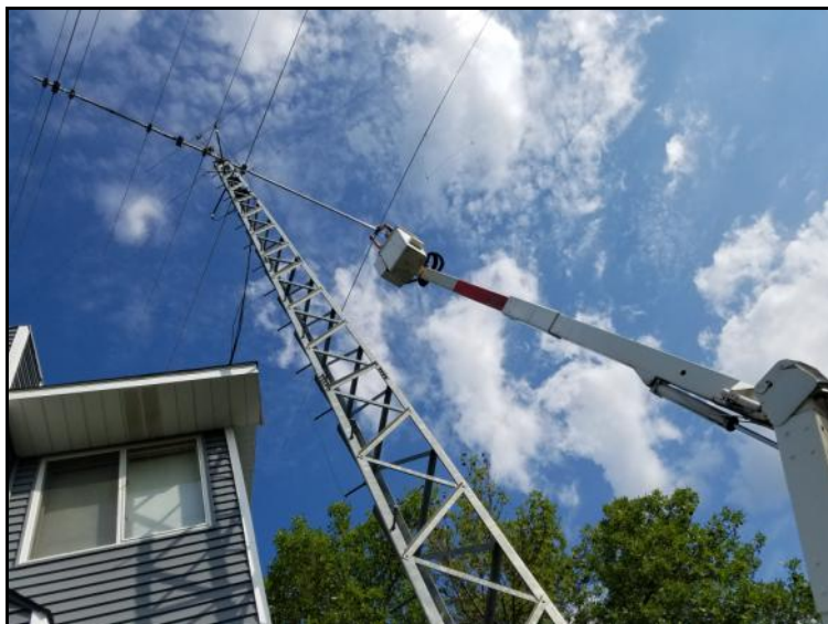
Al, KØAD removing the old 40M Reflector from the C4SXL yagi
